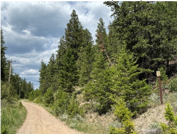
Figure 36: The Camp One Access Road and hydro line beside the reserve (note: eco-reserve sign), June 6, 2025.
