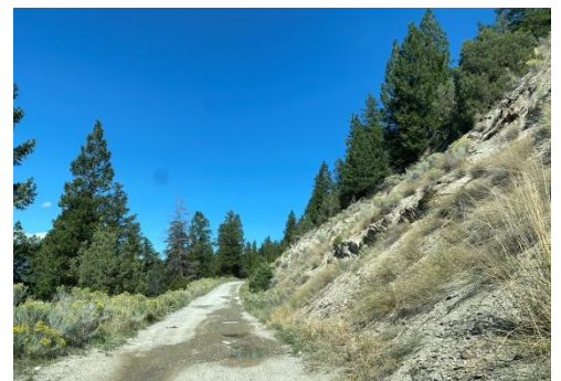
Figure 46. Water running down access road from cold springs in and around the CLER, causing ruts and potholes and depleting the CLER of water.
