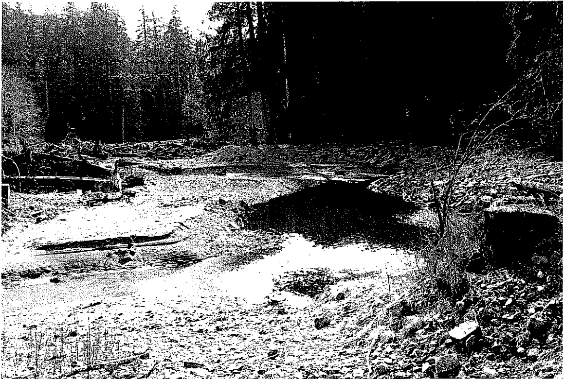
PHOTO 8: MAIN CUTOFF CHANNEL, LOOKING SOUTH ACROSS RIPRAP AND 1987 BERM
