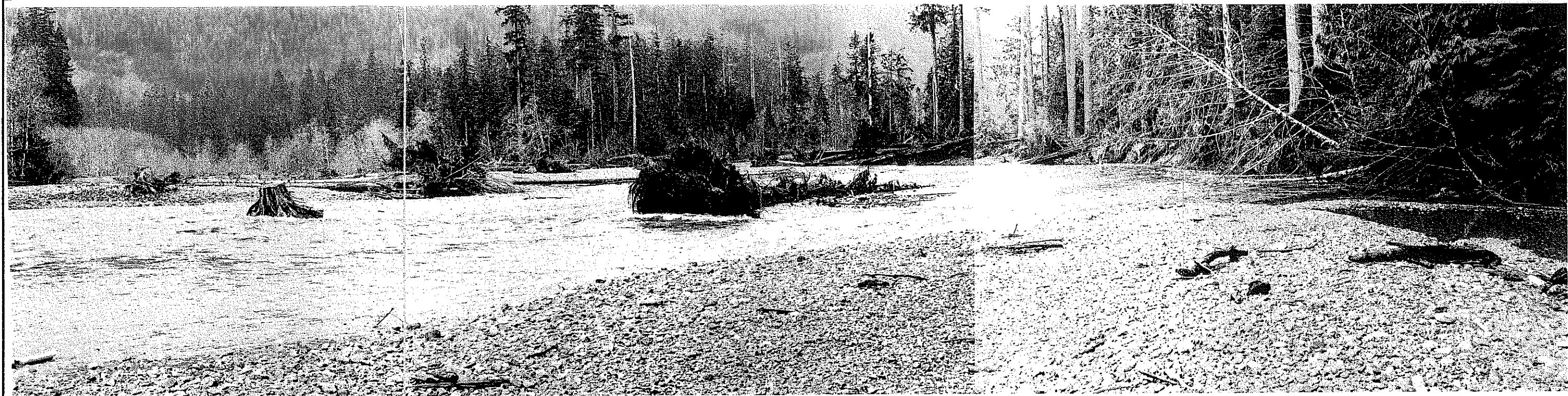
PHOTO 3• VIEW DOWNSTREAM IN NIMPKISH AT NORTH END OF ISLAND
